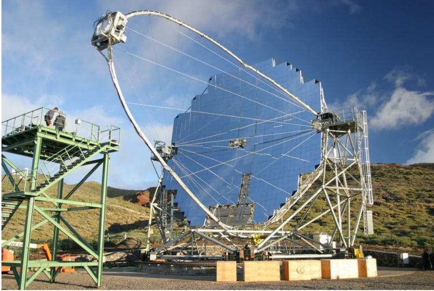
Figure 1. View of the MAGIC telescope right before its inauguration in October 2003. Its 17 m diameter reflector makes it into the largest Imaging Cherenkov Telescope in the world. The main mirror is composed of 940 1 \text{ m}^2 mirror panels that are fully steerable using an active mirror control system.
