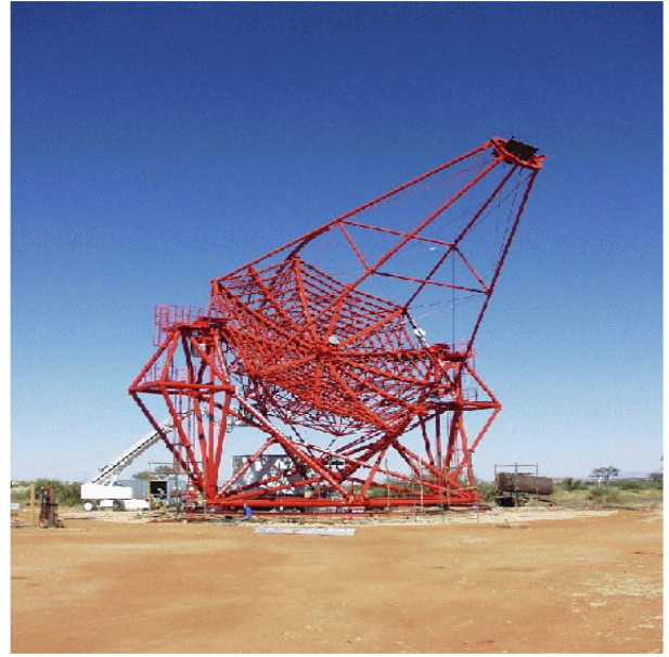
Fig. 24. Steel frame of the first H.E.S.S. telescope. Rotation around the vertical axis is on a circular rail of \sim 15 m diameter.
